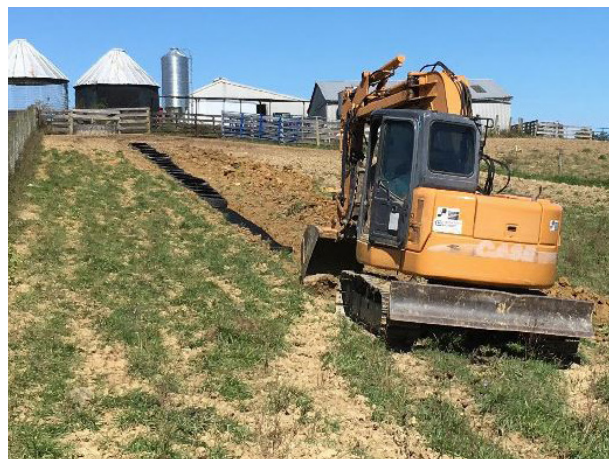
A backhoe cretes a trench for an all weather path.
