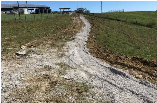
A completed trail leads to water source located on a hill with 30% slopes.
