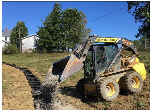
The tread cylinders are filled with rock.
